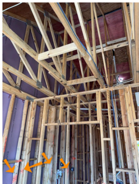
All bowed 2x4's were marked with a 'B' & arrow of direction it needs to move.
