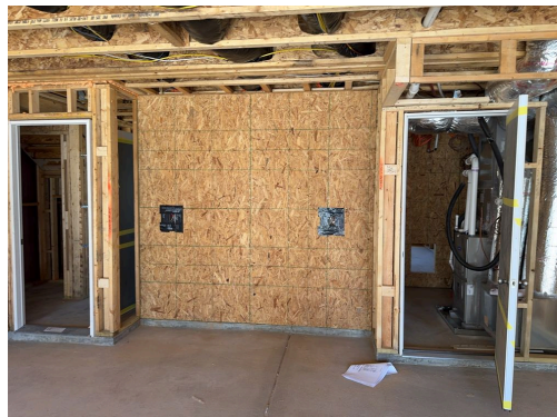
Left – living space, right – utility room
