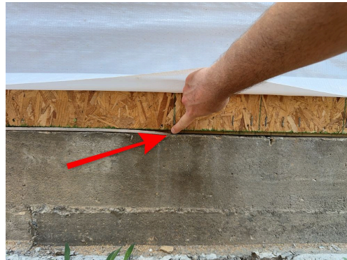
White foam sill sealer ripped where
