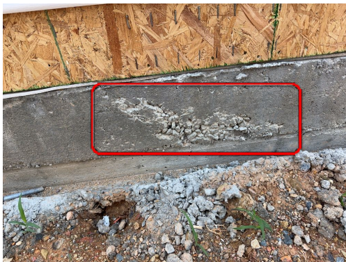
Honeycombing on exterior foundation wall
